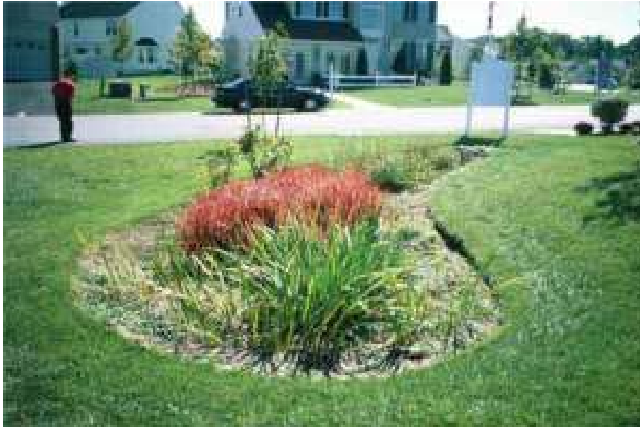
A Rain Garden created to infiltrate stormwater
