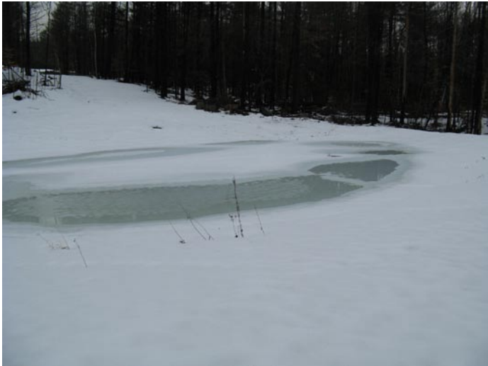
Photograph of same wet pond taken on March 11, 2009 during rain event. Note the lack of freeboard on standpipe resulting in direct discharge of runoff during rain event show in adjacent photograph.
