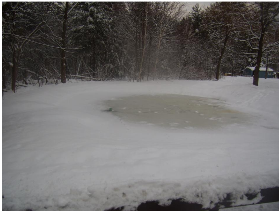
Photograph of wet pond constructed at the Blue Lagoon Resort. Note the standpipe on the left side of the pond and the ice elevation which reduces the ability for stormwater management.
