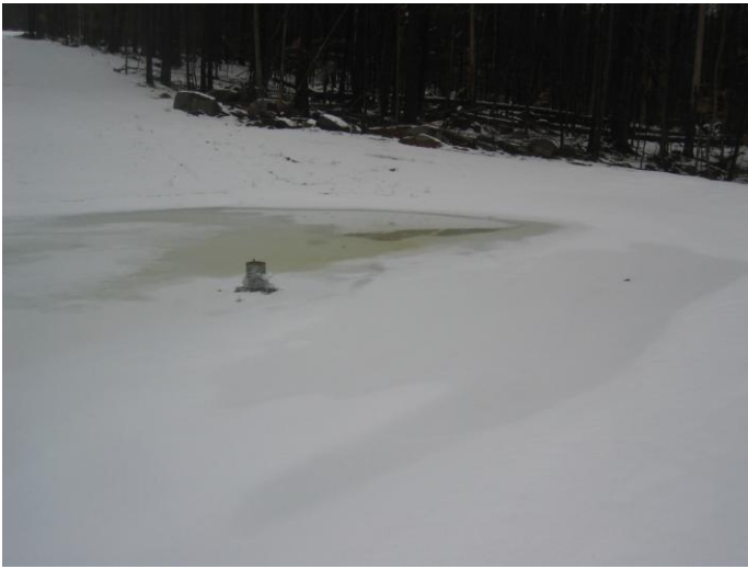
Photograph of wet pond - Town of Hague subdivision taken on January 30, 2008. Note the freeboard height of the standpipe above the ice elevation.
